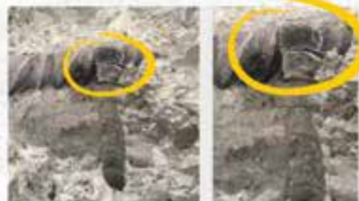
Detail of the concrete and the rebar tapped by CONCRETO® screw
